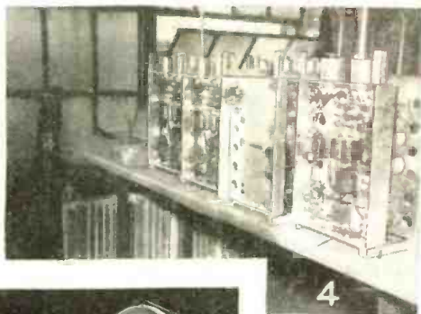
3 Chassis of the 21-tube television and sound receiver.
